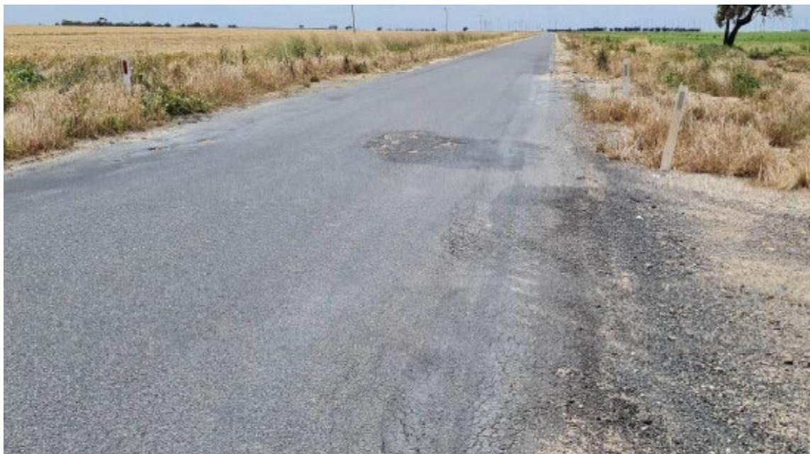
Figure 2.0 – Typical condition of Dimboola-Minyip Road taken following damage in 2022.
