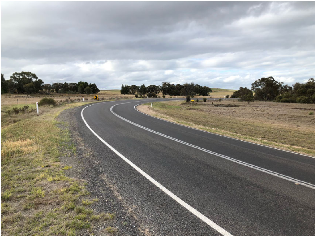
Looking Left from proposed new access location
