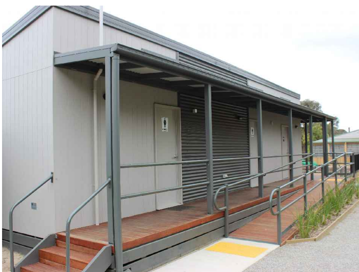
Amenities Block - including all abilities access camp
