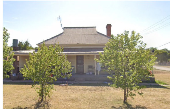
PROPOSED SITE NO.6 BELL ST NHILL SINGLE STOREY WEATHERBOARD CLADDING METAL SHEET ROOF
