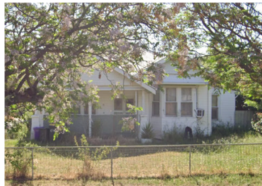
6 GOLDSWORTHY ST SINGLE STOREY WEATHERBOARD CLADDING METAL SHEET ROOF
