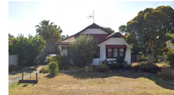
8 GOLDSWORTHY ST SINGLE STOREY WEATHERBOARD CLADDING METAL SHEET ROOF
