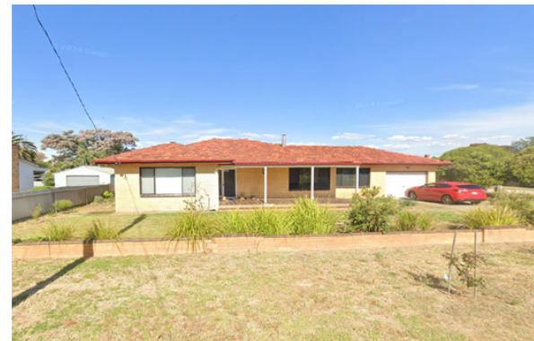
5 GOLDSWORTHY ST BRICK VENEER TILED ROOF
