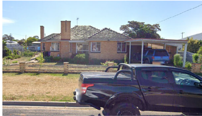
NEIGHBOURING SITE NO.4 BELL ST BRICK VENEER TILED ROOF
