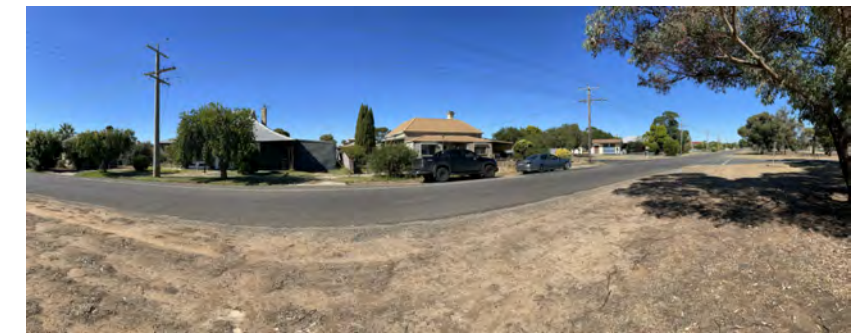
STREET VIEW OF NELSON STREET
