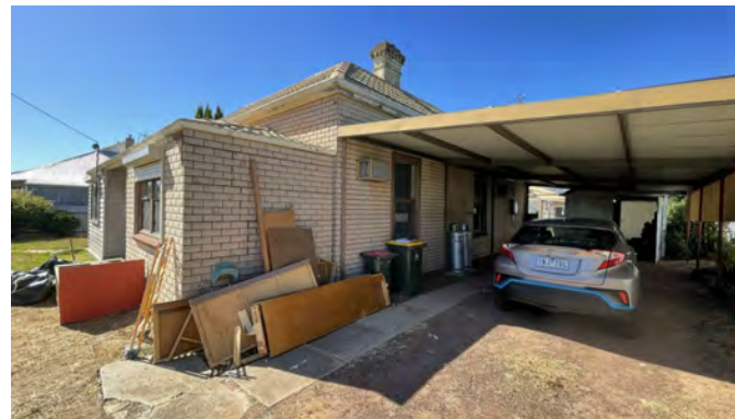
CARPORT OF EXISTING DWELLING
