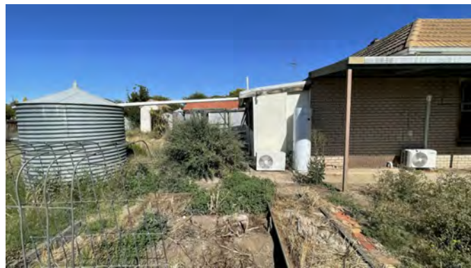
REAR OF EXISTING VERANDAH AND WATER TANK
