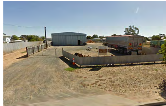
NO. 19-21 ROCKLEY STREET (ADJACENT SITE) EXISTING SHED
