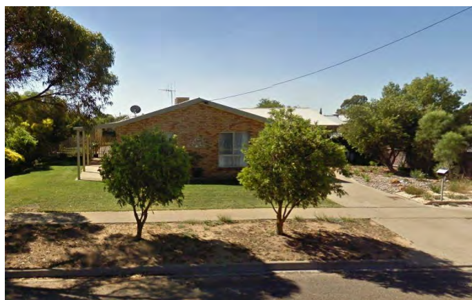
NO. 36 LEAHY STREET (ADJACENT SITE) EXISTING SINGLE STOREY DWELLING BRICK AND TIN ROOF
