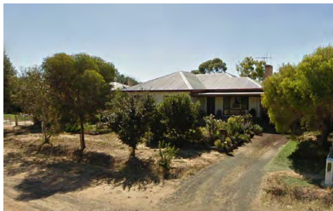
NO. 44 LEAHY STREET (ADJOINING SITE) EXISTING SINGLE STOREY DWELLING WEATHERBOARD AND TIN ROOF
