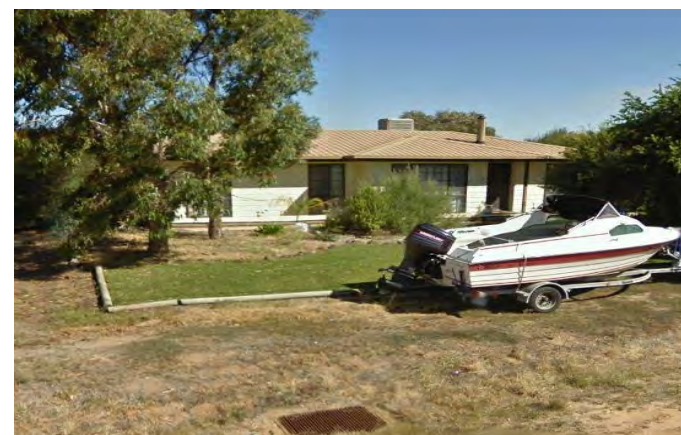
NO. 57 LEAHY STREET (OPPOSITE SITE) EXISTING SINGLE STOREY DWELLING WEATHERBOARD AND TIN ROOF
