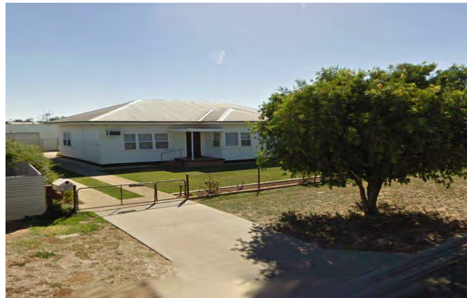
NO. 8 RUSSELL STREET (ADJOINING SITE) EXISTING SINGLE STOREY DWELLING WEATHERBOARD AND TIN ROOF
