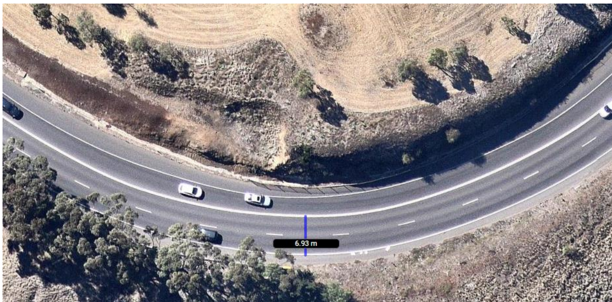
Figure 16 – Aerial imagery measurement of seal width on curved section of road
