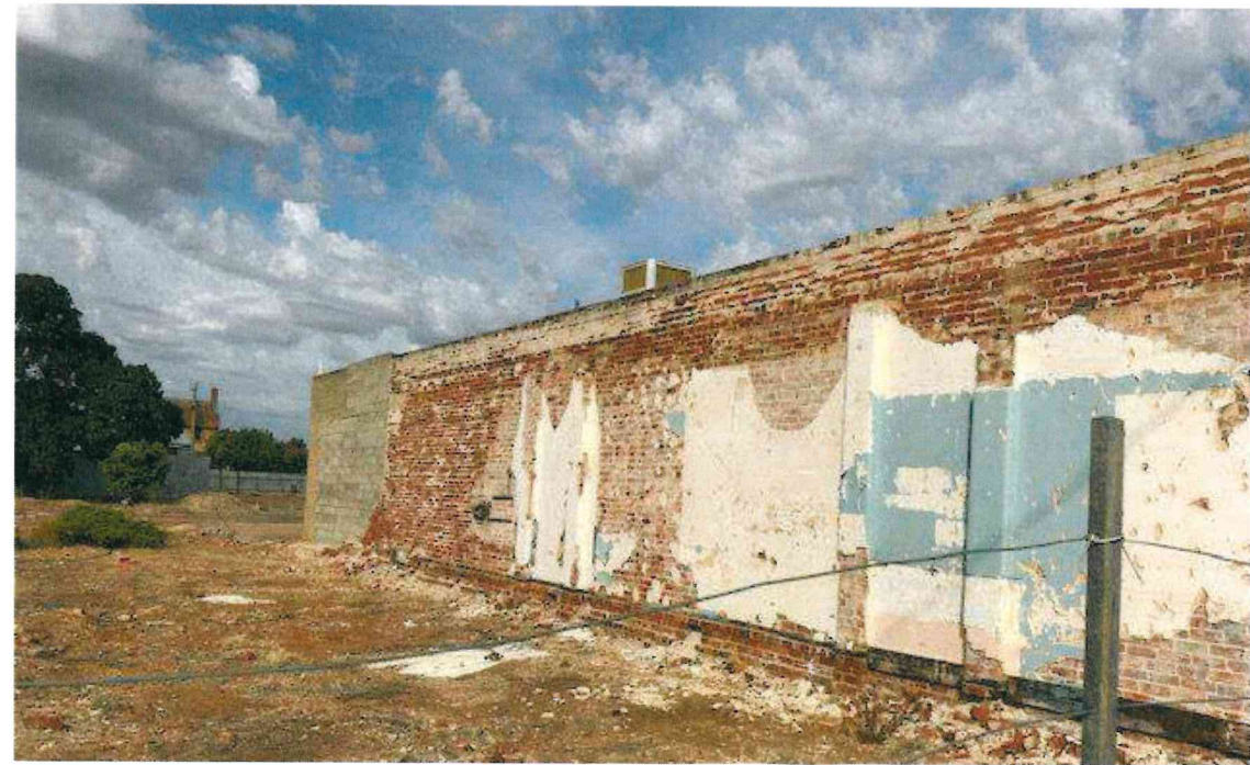
VIEW OF EXISTING HISTORIC BRICK BOUNDARY WALL TO BE RETAINED
