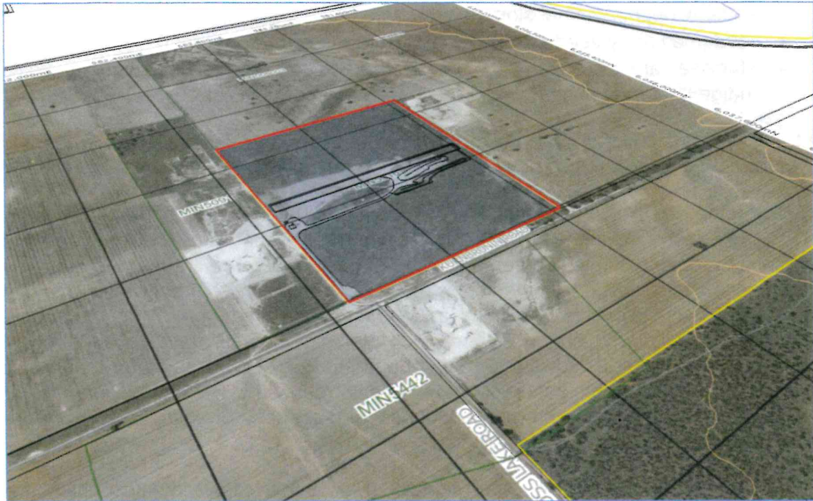
Figure 5.1: Gould's Pit – Current Appearance
