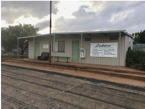
Existing netball clubrooms above
