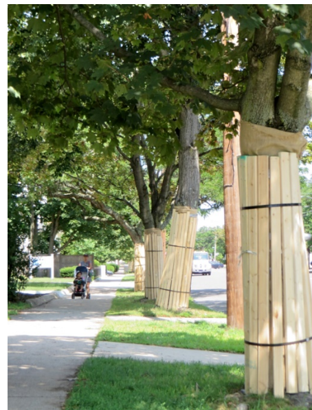
Figure 7: photo of trunk protection
