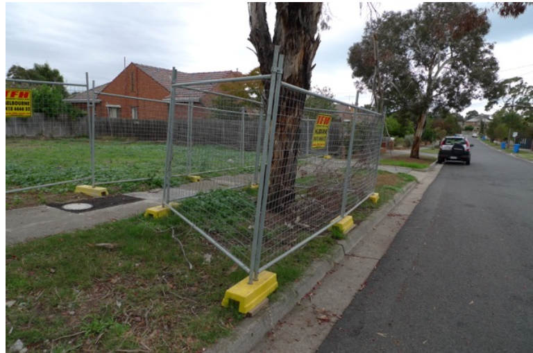
Figure 6: Photograph above left - example of signage for TPZ. Photograph above right - example of appropriate TPZ fencing around a street tree.
