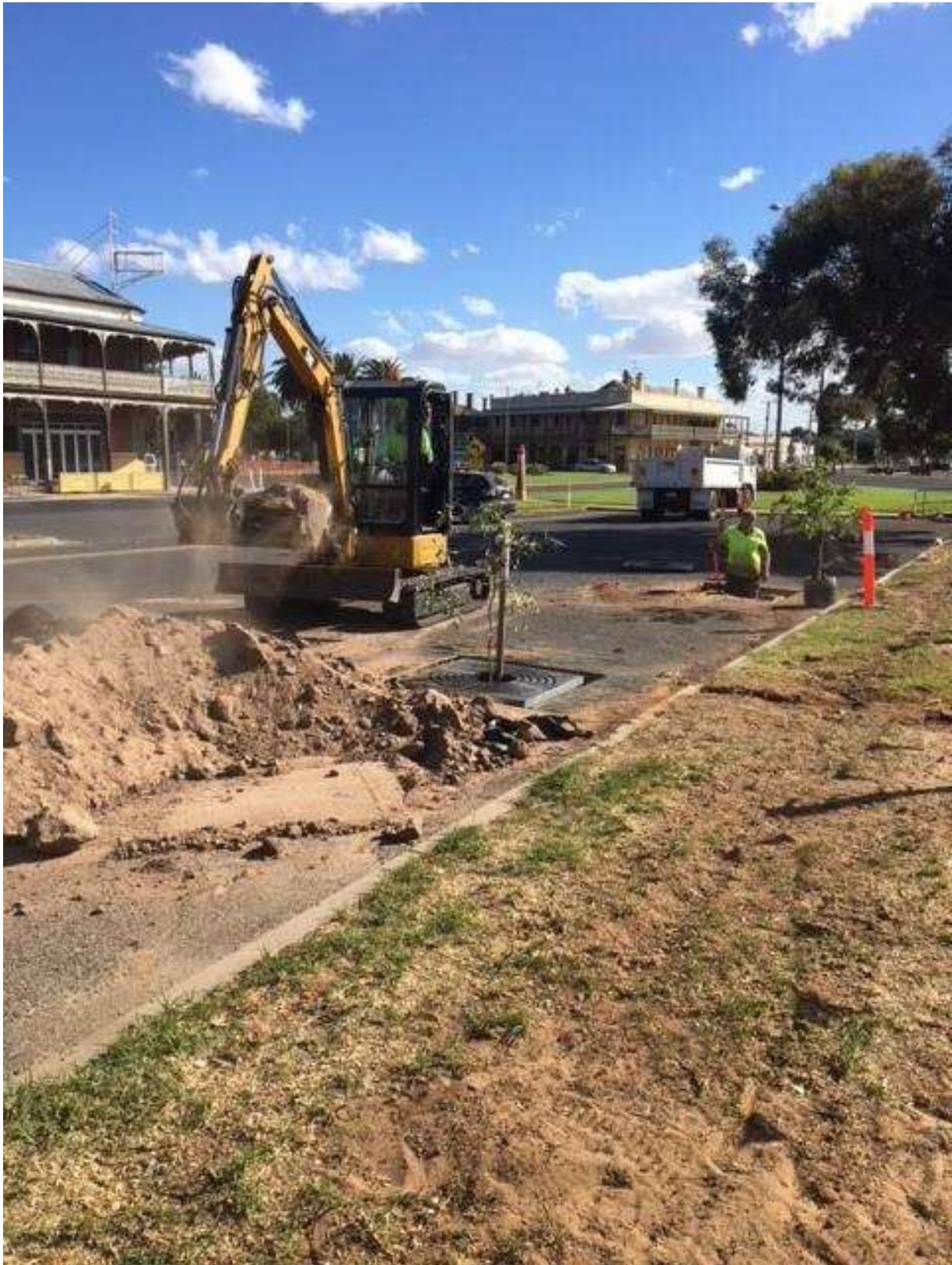
Nhill's Commercial Carpark upgrade
