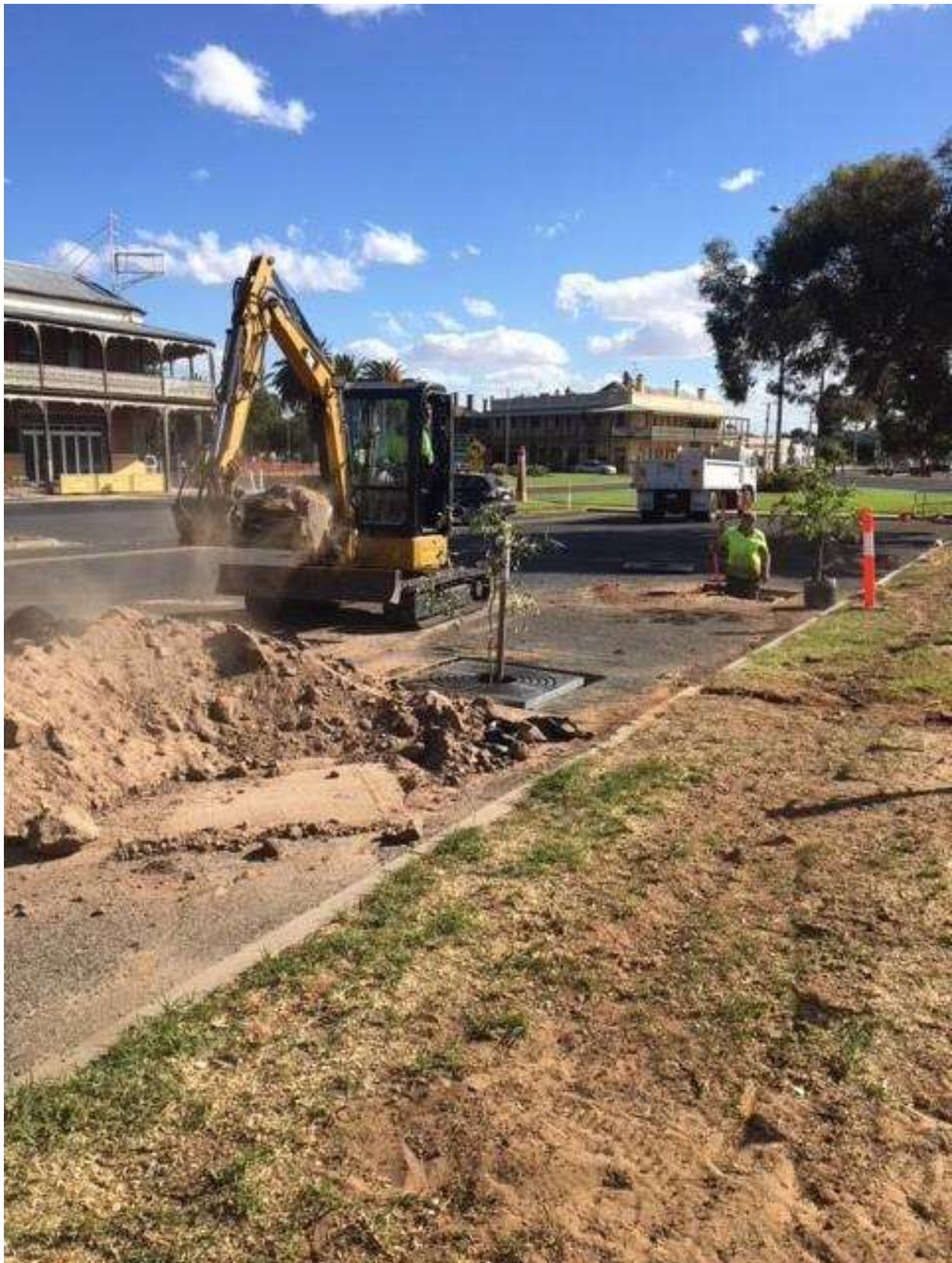
Nhill's Commercial Carpark upgrade
