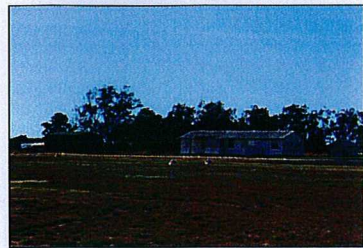
Photo 110825 04: View from airfield towards the Flight Office and the Freeman Aerial Services shed.
