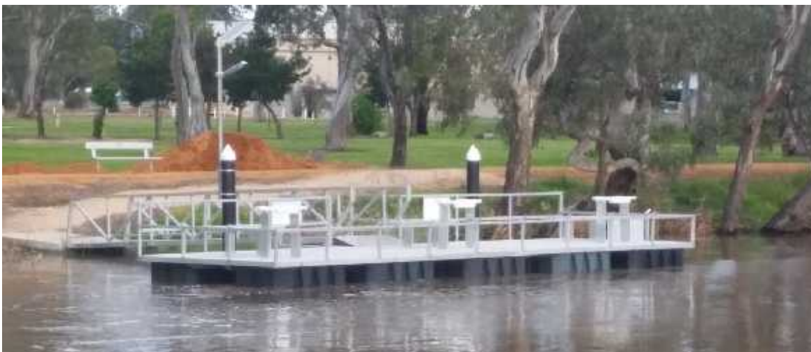
Fishing pontoon at Dimboola, similar to what is proposed for installation at Nhill Lake
