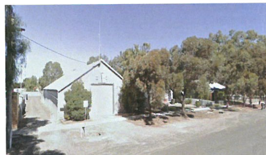
Figure 16 - Current SES building from Lochiel Street
