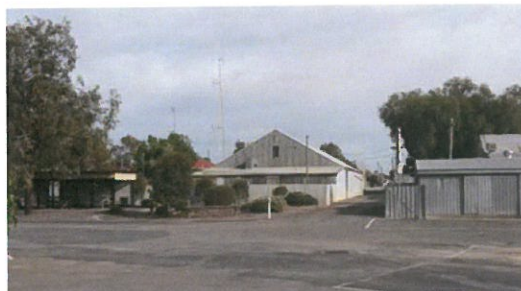
Figure 14 - Rear of current SES building in from library car park
