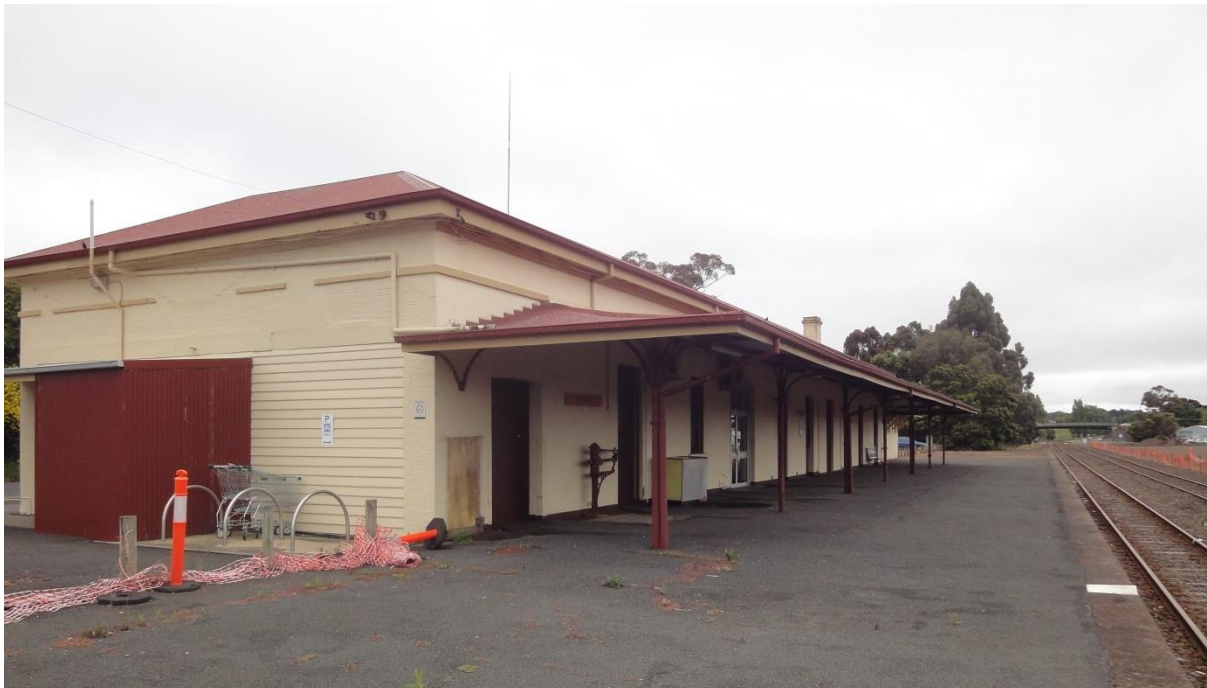
Figure 23: Hamilton station building and platform
