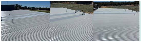
Contractors have recently completed the installation of a new roof on the football changerooms at the Rainbow Recreation Reserve. The old roof has been replaced due to a large number of ongoing leaks.
